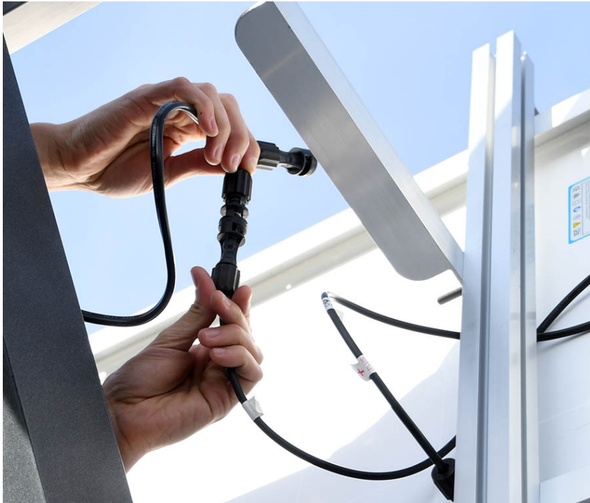
FIGURE 4-4 Connect Solar Cable to Panel
