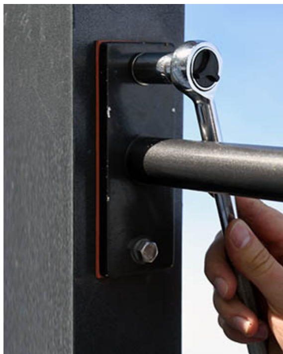
FIGURE 4-10 Weather Arm Bolted to the Pole
