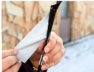
FIGURE 3-9 CBL222-20 Routing with Fish Tape
