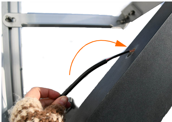
FIGURE 4-2 Feed Cable Down Pole
